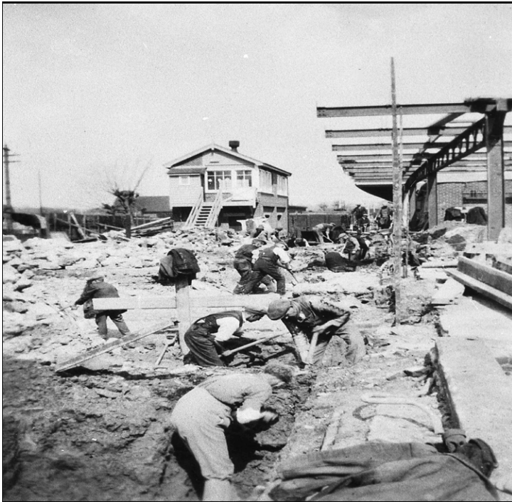
Re-building Haywards Heath station in 1932 prior to electrification of the line
