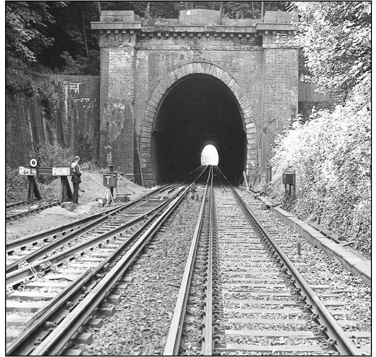
Looking south through Haywards Heath (Folly Hill) tunnel
